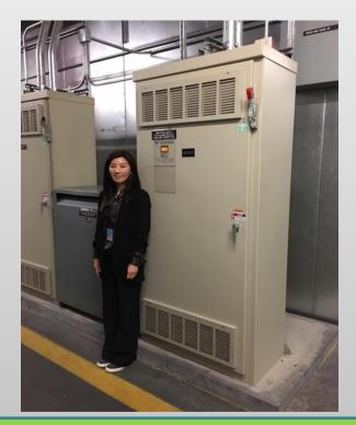
In this picture a Variable Frequency Drive powering a Main Terminal Air Handling Unit fan running at 350 Horsepower
